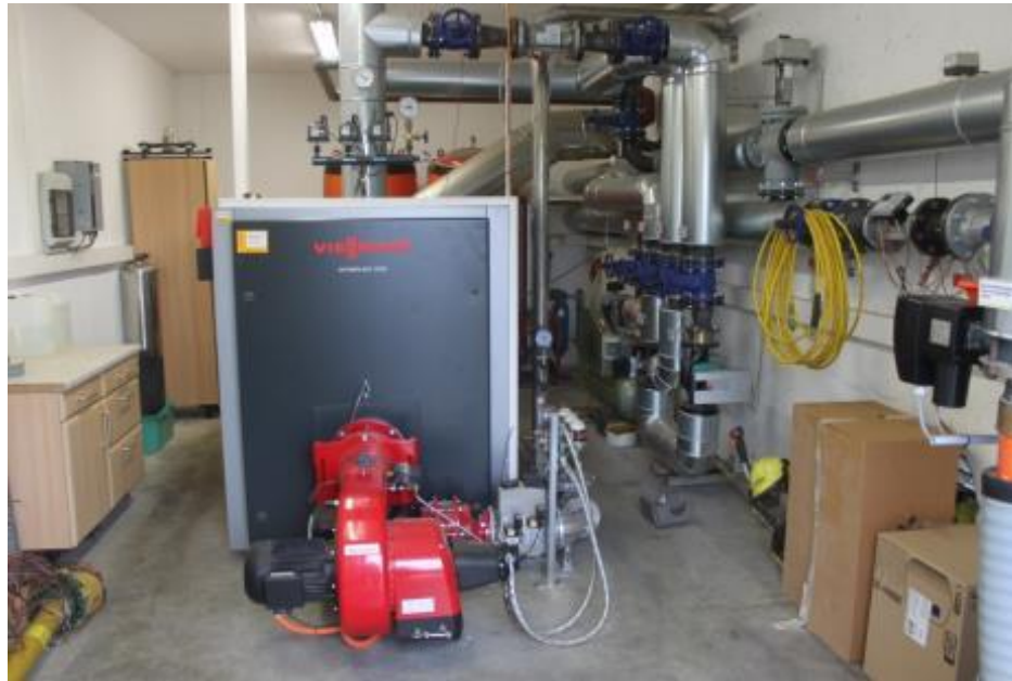
Peak load boiler for fossil heating oil at a biogas plant in Germany (Source: Rutz D.)
