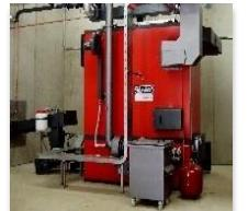
Hot water boiler ( $> 110 \text{ }^{\circ}\text{C}$ )
