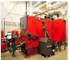
Warm water boiler ( $\leq 110 \text{ }^{\circ}\text{C}$ )
