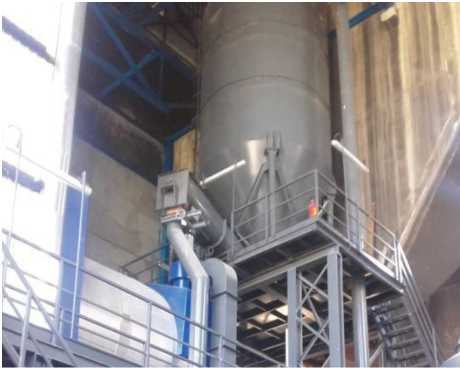
Figure 8 Biomass depot before boiler in Sremska Mitrovica district heating plant
