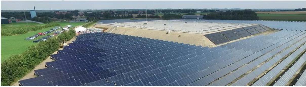
Figure 3: The new solar system established in 2015 including solar voltaic panels on the south side of the seasonal pit storage, picture by Gram Fjernvarme
