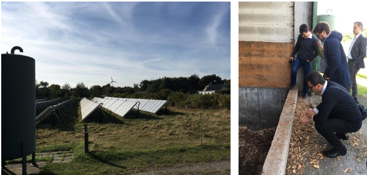
Figure 6: Photos from Nordby/Mårup Varmeværk with solar DH and biomass (L. Laurberg Jensen)
