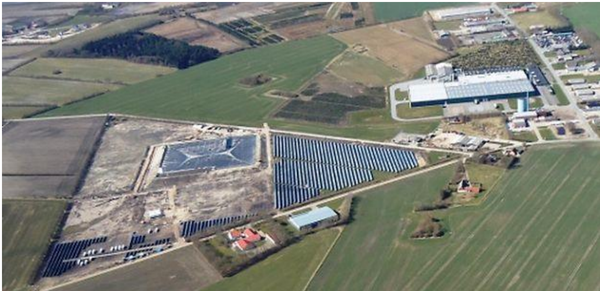
Figure 2: The seasonal pit storage and the solar field under establishment. To the right is the existing 10,000 m 2 and at left and front is seen the area where the new solar panels installed together with the seasonal pit storage, picture by Gram Fjernvarme
