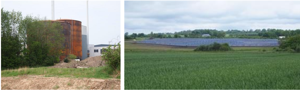
Figure 5: Right: The two new accumulation tanks in relation to the solar field under construction, right: view of the solar field ( http://www.jelling-varmevaerk.dk/solvarme ).
