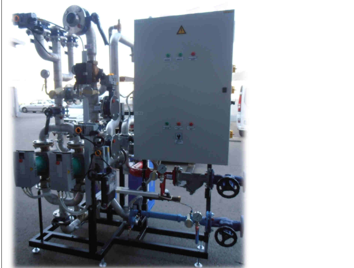
Picture 4: Distributor / collector for heating
