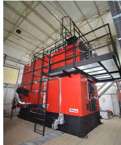
Steam boiler 3 MW
