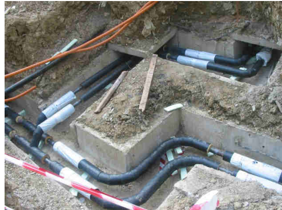
Installation of pre-insulated pipes PURLEN-A
