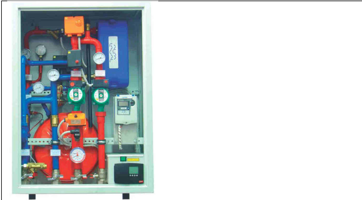
Picture 3: Compact heating sub-station for preparation of sanitary hot water
