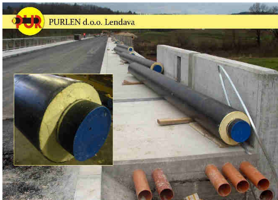
Pre-insulated pipes – duktil
