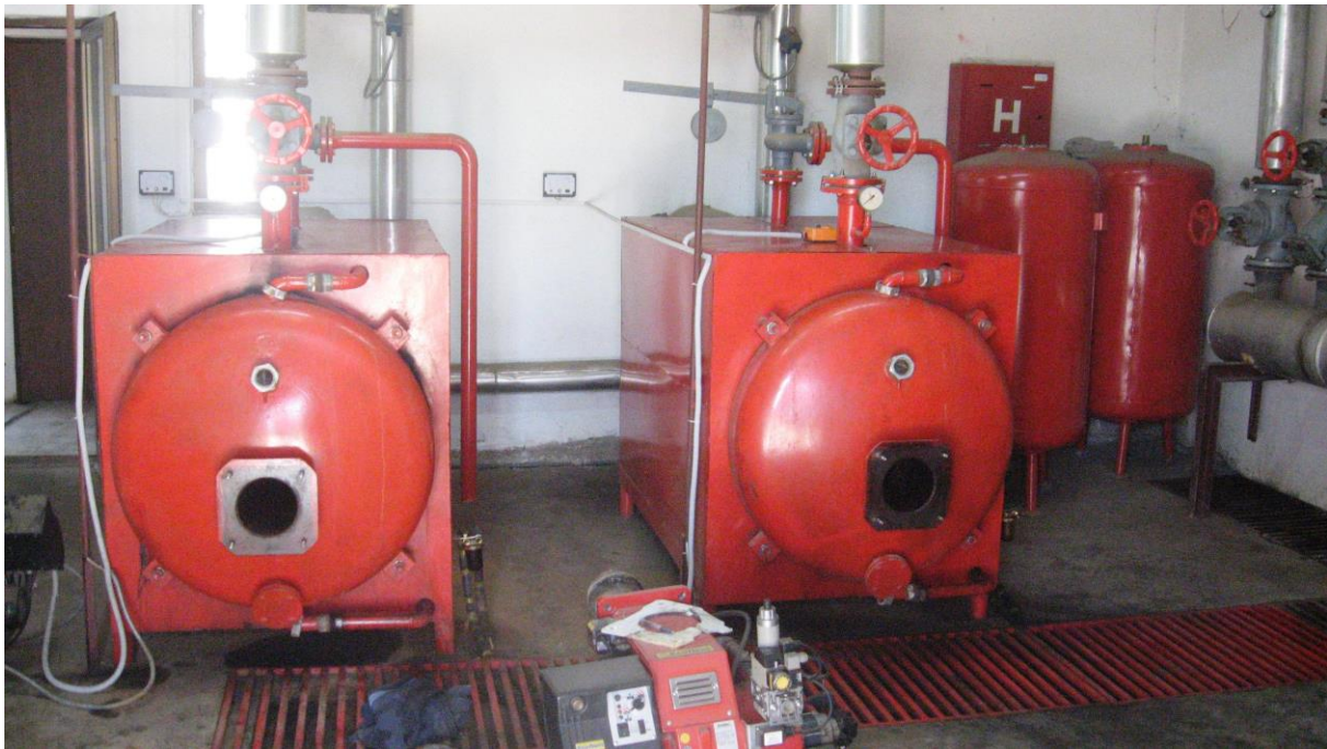
Figure 8: Two fuel oil boilers inside of the boiler room (Source: Slobodan Jerotić)
