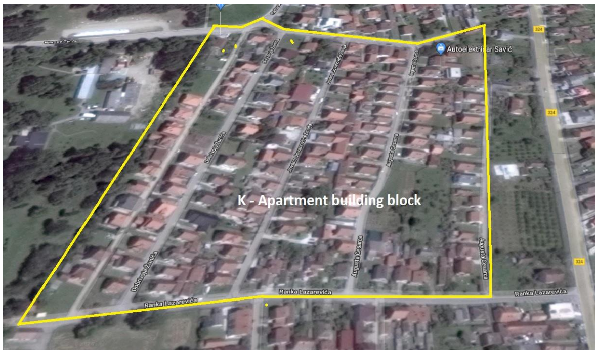
Figure 6: Apartment building block K (Source: Google maps)
