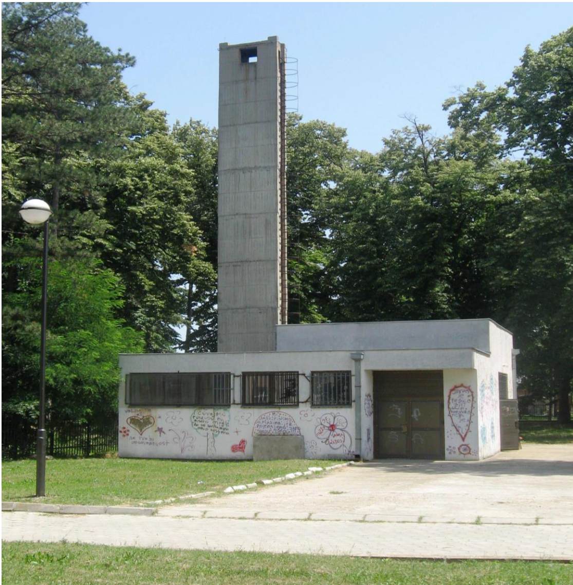
Figure 7: Existing boiler room at location "LETNJKOVAC" (Source: Slobodan Jerotić)
