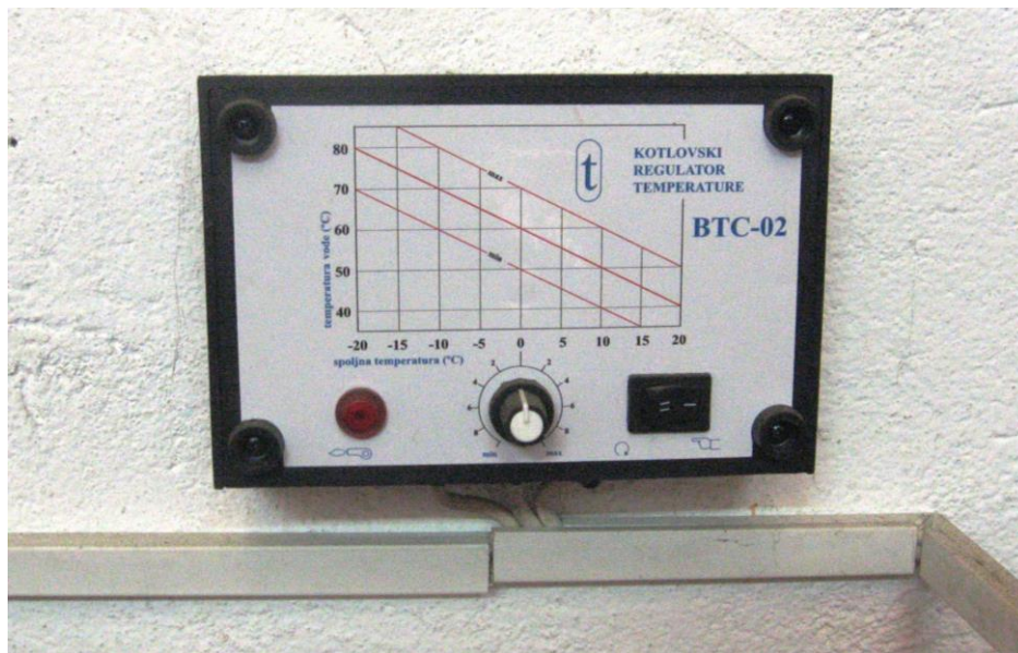
Figure 9: Boiler controller (Source: Slobodan Jerotić)
