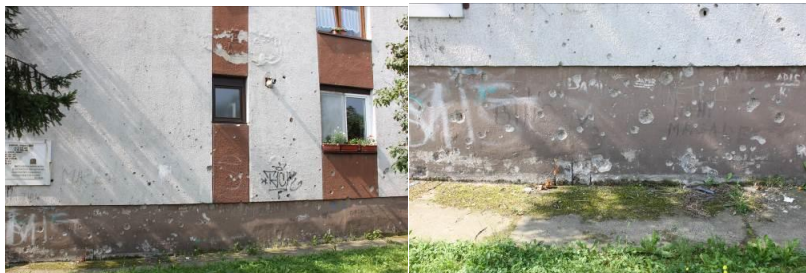
Figure 8: Damage on most of buildings remained from war time
