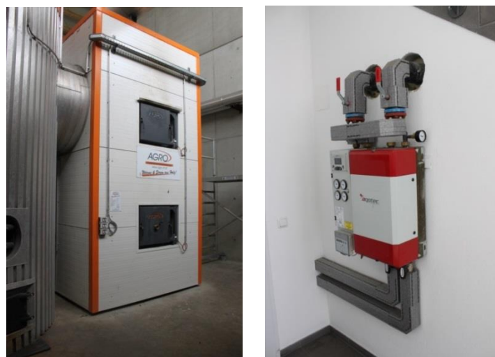
Figure 16: Woodchip boiler (left) and heat transfer station (heat exchanger) used in the households (right) of the heating grid in Grassau (Source: D. Rutz, WIP)
