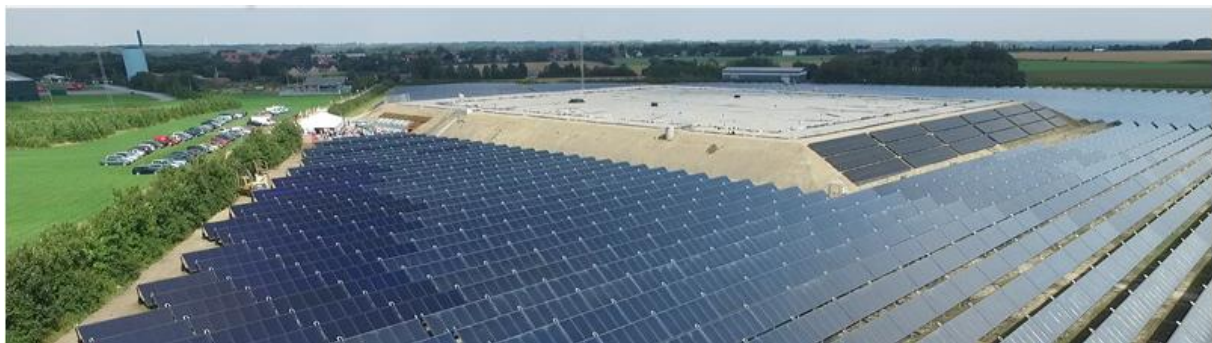
Figure 5: The new solar system established in 2015 including solar voltaic panels on the south side of the seasonal pit storage, picture by Gram Fjernvarme
