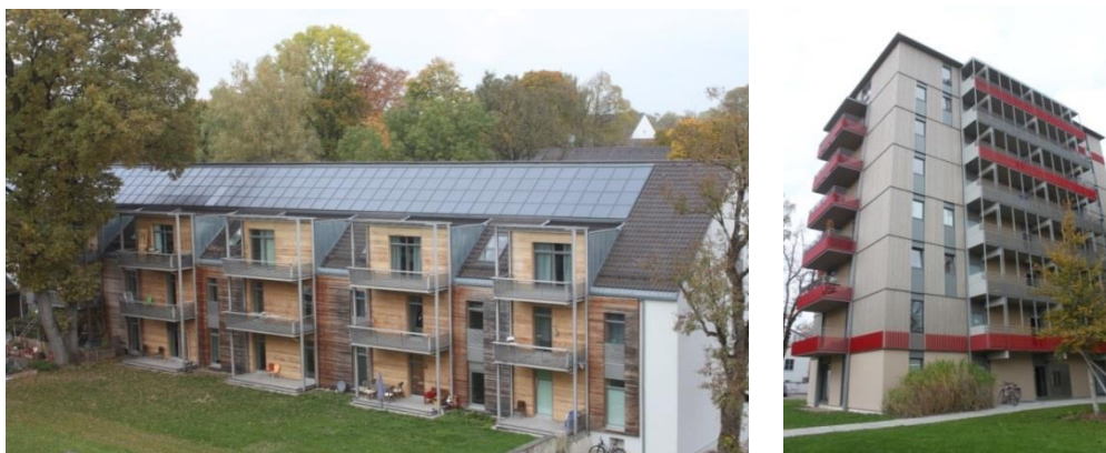
Figure 18: Solar collectors (left) and 8-floor wood house in Bad Aibling (Source: D. Rutz, WIP)
