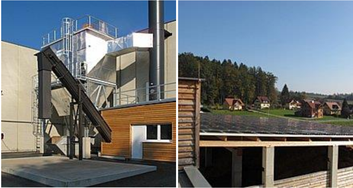
Figure 26: Exhaust gas cleaning at the biomass plant Stainz with an electrostatic filter; Photovoltaic modules with 257 kW p on the roof of the biomass storage (Photos by: nahwaerme.at)
