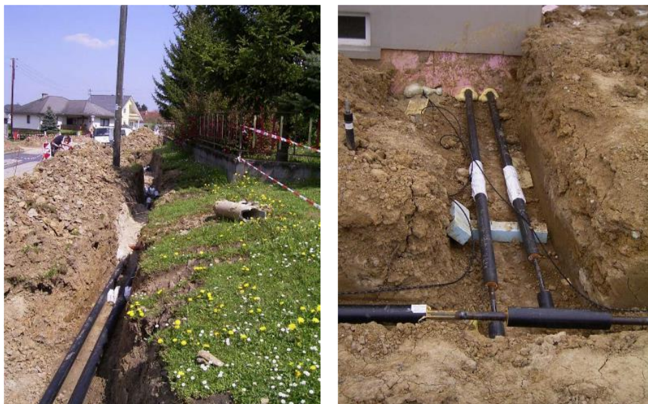
Figure 22: District heating pipes while installing the grid; Connection to the households (Source: Güssinger Fernwärme GmbH)
