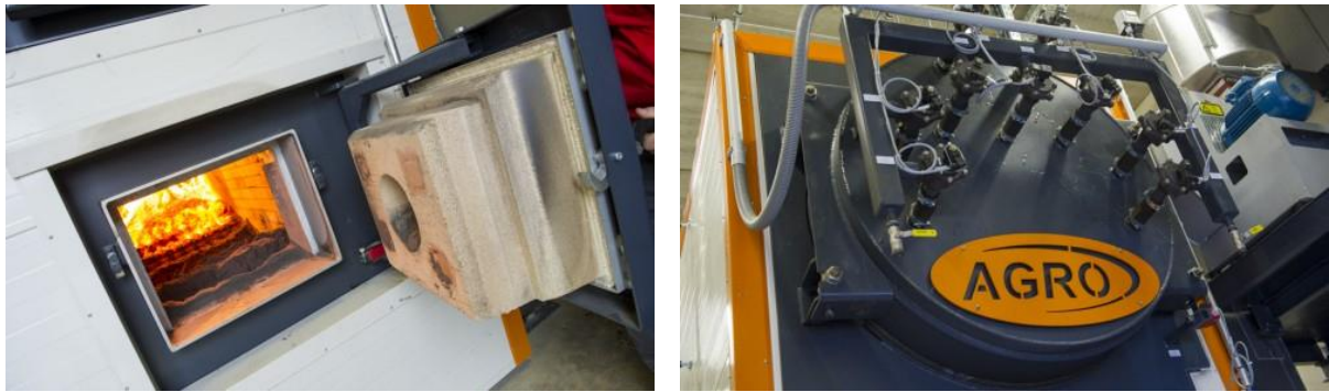
Figure 28: Grate of the biomass boiler; Biomass boiler with cleaning unit (Source: http://holzdiesonne.net/hsh-nahw%C3%A4rme/nahw%C3%A4rme-lavam%C3%BCnd/ )
