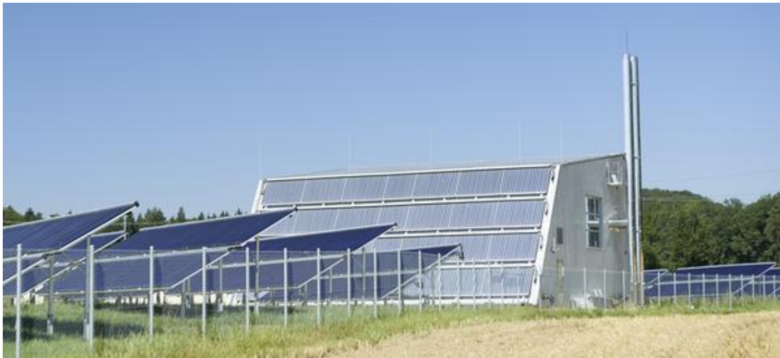
Figure 13: 1,000 m 2 vacuum tube solar collectors of the bioenergy village Büsingen (Source: Solarcomplex)
