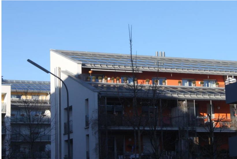
Figure 10: Solar collectors on the rooftop of the apartment houses at “Am Ackermannbogen” (Source: D. Rutz, WIP)
