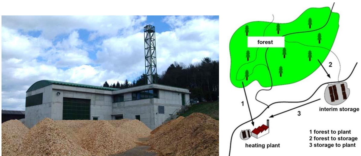
Figure 23: Biomass heating plant with 1MW biomass boiler and 1.3 MW oil peak load boiler (Source: EEE GmbH); Concept for mobilizing unused resources from local forests in Güttenbach with an interim storage
