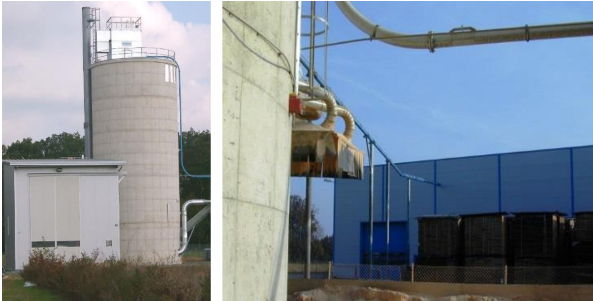
Figure 24: Heating plant II in Güssing to fire saw dust for heat production (Source: EEE GmbH); The storage is provided with saw dust from 2 wood floor companies (Source: EEE GmbH)
