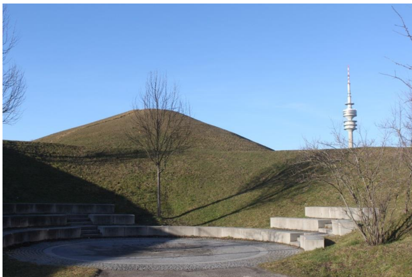
Figure 11: Seasonal storage tank covered with soil and well-integrated in the urban planning at “Am Ackermannbogen” (Source: D. Rutz, WIP)
