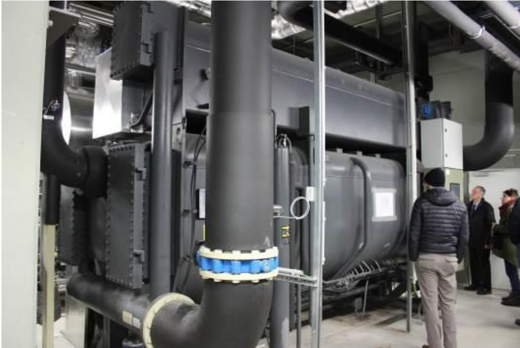
Figure 8: Steam double effect absorption chiller
