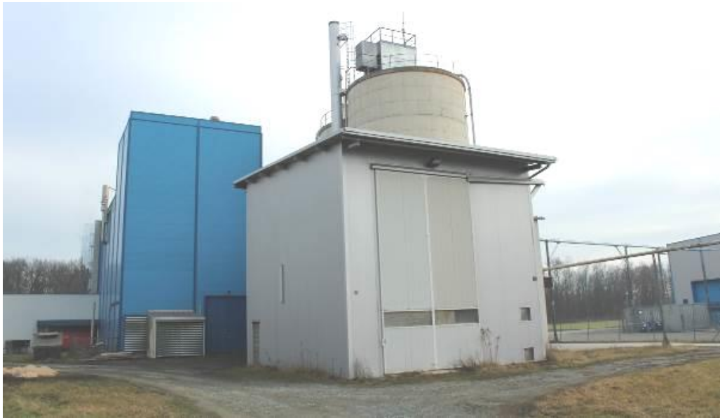
Figure 15: District heating plant
