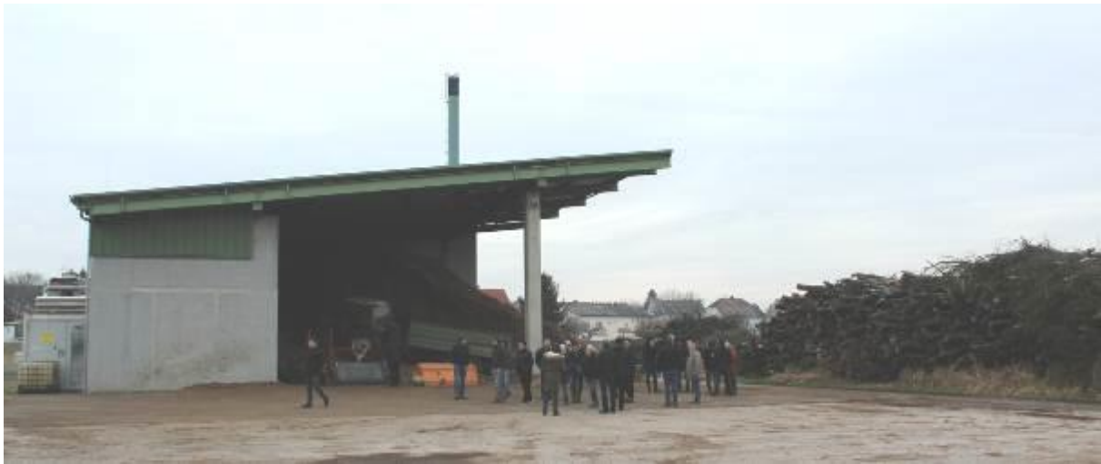
Figure 10: Biomass heating plant in St. Michael
