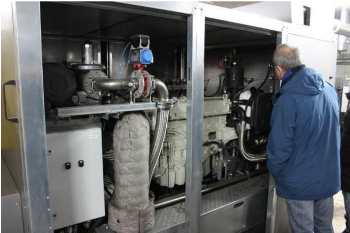
Figure 2: Wood gas engine
