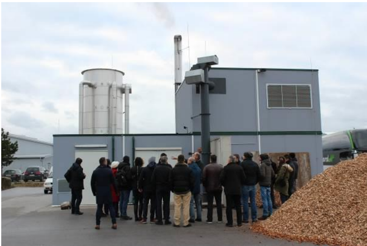
Figure 5: Biomass heating plant in Wöllersdorf
