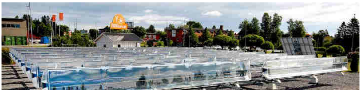
Ground mounted field with a secondary loop connection, in Härnösand, Sweden. 200 m 2
