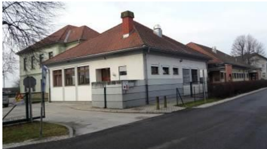
Figure 3: Ground school Cven
